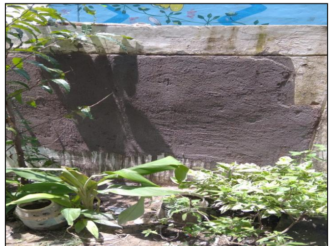
NG-Khudmuda-05_Durg inside repair after
