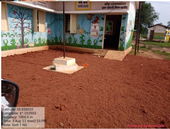
Dumping of soil_Sorli_Balod
